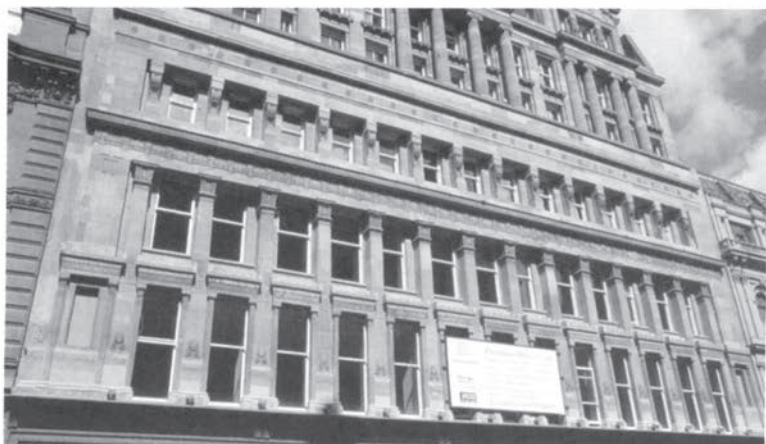
The Grosvenor Building, Gordon Street (Alexander Thomson, 1859-61, rebuilt 1866 – the addition, above Thomson's topmost cornice, by J.H. Craigie, 1907).
