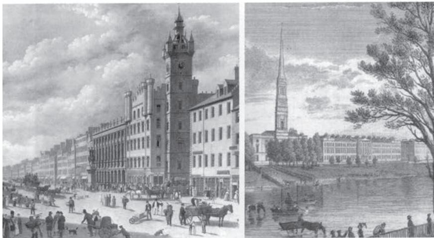
Left: Trongate and Argyle Street, with the Tolbooth steeple, Tolbooth and beyond them the Tontine Hotel. Of the three, only the steeple survives. Painting by John Knox, c. 1820. Right: Carlton Place (Peter Nicholson, 1813-18), with Gorbals Parish Church (David Hamilton, 1806-10, demolished 1973).
